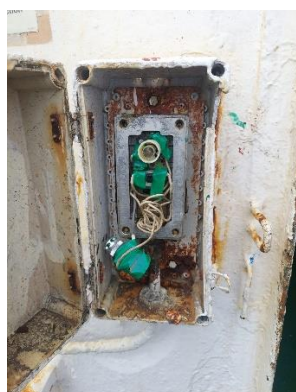
Sludge P/P Remote St./Stp. Switch Defective
