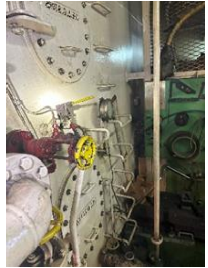
Quick closing valve spindle missing
