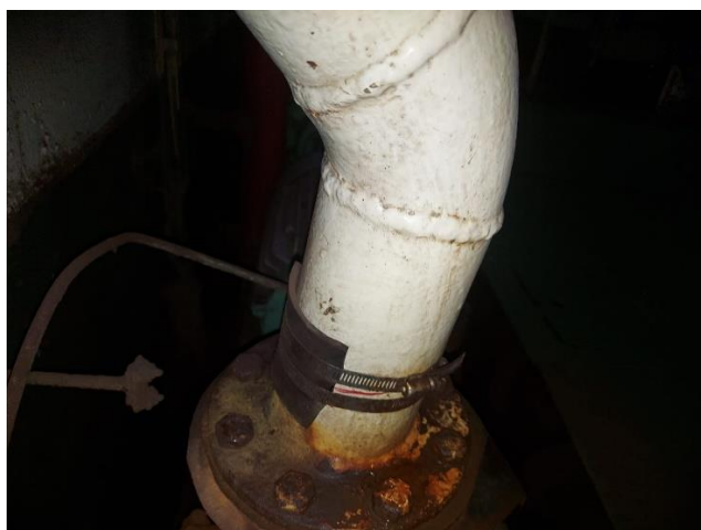
Temporary repairs on S/W Pipeline
