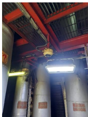
Damaged Fire Detector
